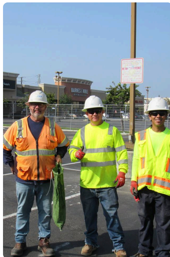
CES field team on a commercial remediation site
